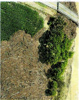
"Slash" knocked out Hikurangi Bridge, north of Tolaga Bay, in this week's storms.
